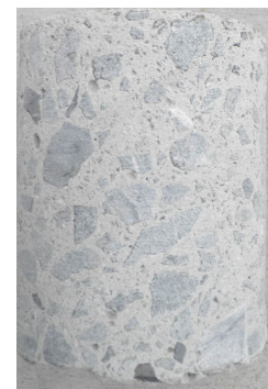
View of core removed for diagnosis.
